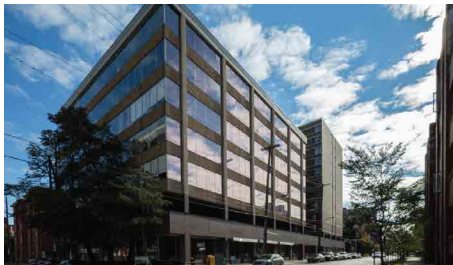
225 Metcalfe Street Office Units: 850 - 7,100 SF
