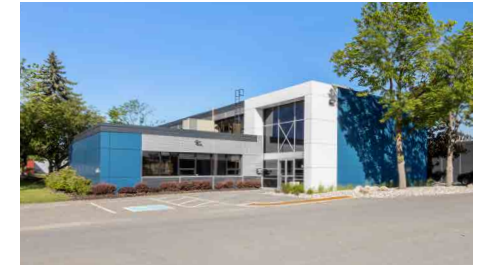
1891 Robertson Road Office Space: 13,043 - 18,657 SF
